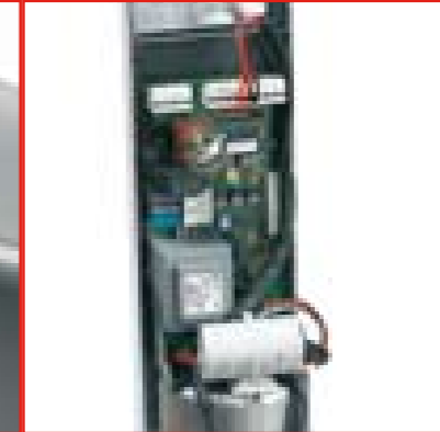
Housing of the control unit
